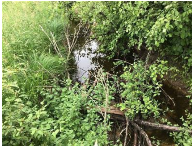
Upstream from structure
