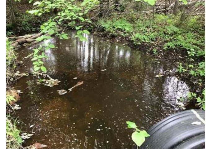
Downstream from structure
