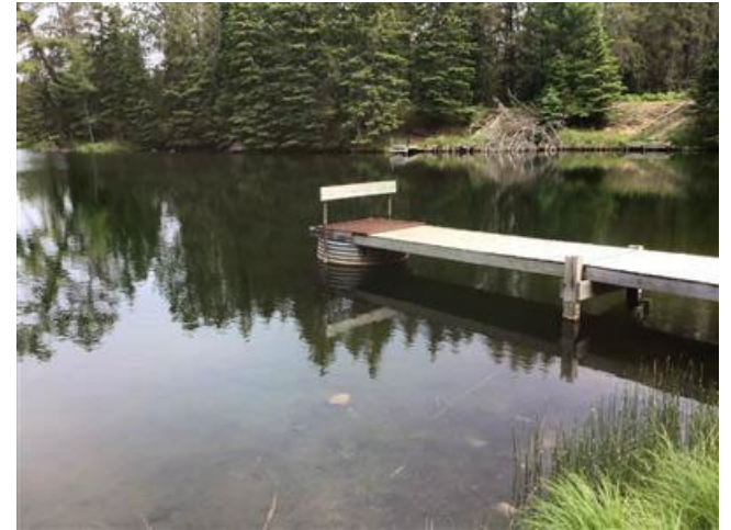
Upstream from structure
