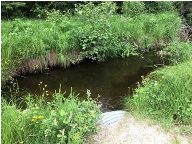
Upstream from structure
