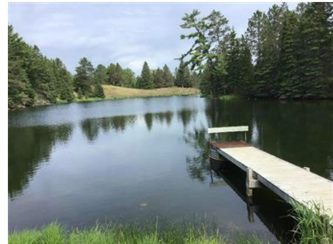
Structure inlet projecting from pond
