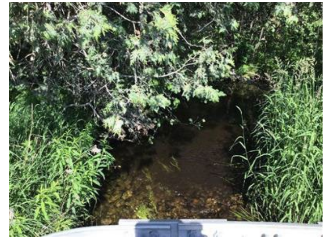
Downstream from structure
