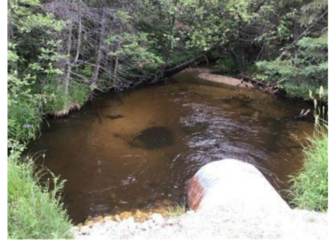
Downstream from structure
