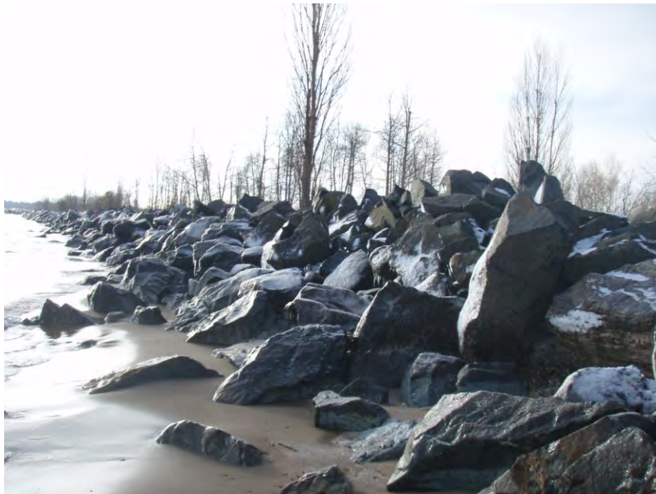
Figure 1.3 Lakeshore Boulevard Stone Revetment
