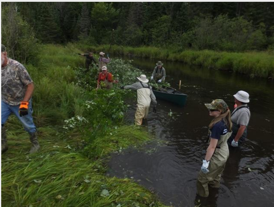
Constructing brush bundles
