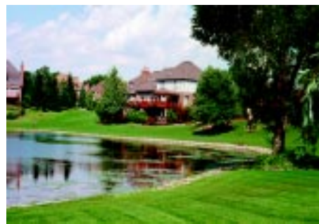
Wet Detention Basin
