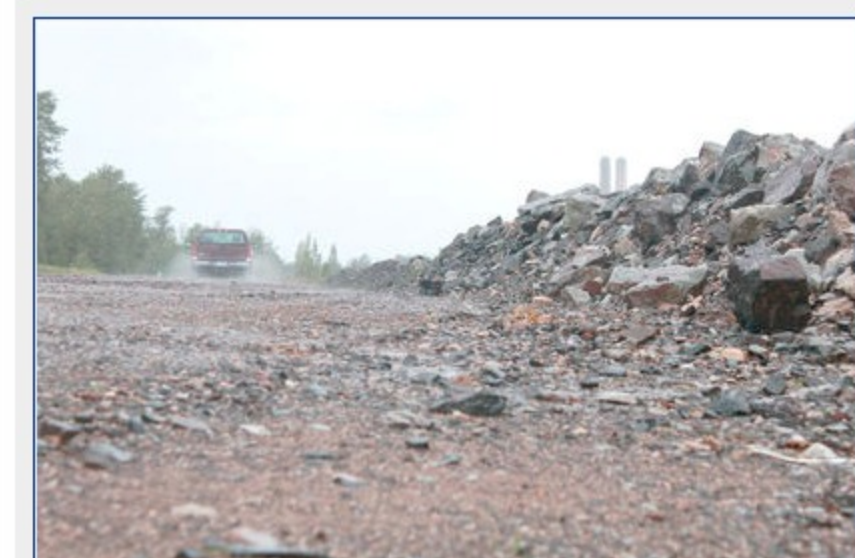
A half-mile stretch of rock rip-rap along Lakeshore Boule...
